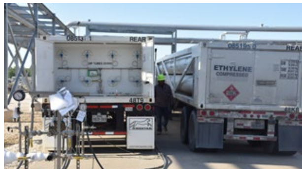
Turnkey supply for pipeline curtailment
