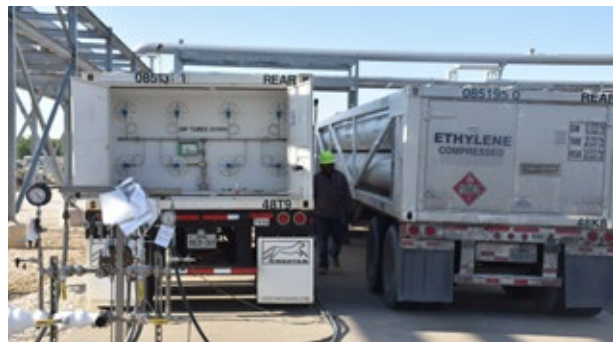
Turnkey supply for pipeline curtailment
