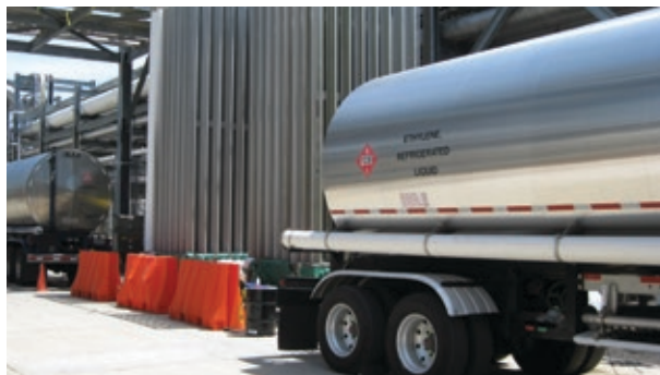
Interim gas flow outages utilizing 2-80 K vaporizers
