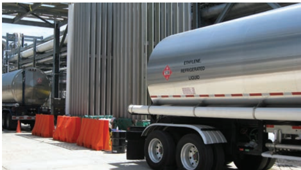
Interim gas flow outages utilizing 2-80 K vaporizers
