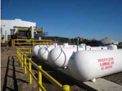
4-1,000 GALLON TANKS INSTALLED AND PIPED INTO PLANT
